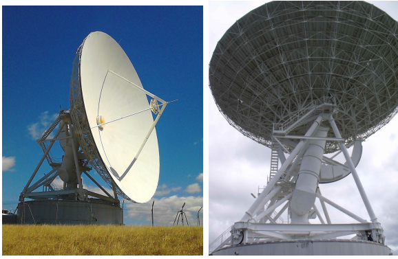
Figure 3. Photos of the 30-m antenna (after cleaning). Images courtesy of Stuart Weston
